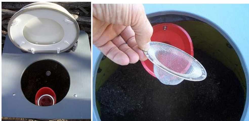
Figure 4-6 Urine diversion system [22]
